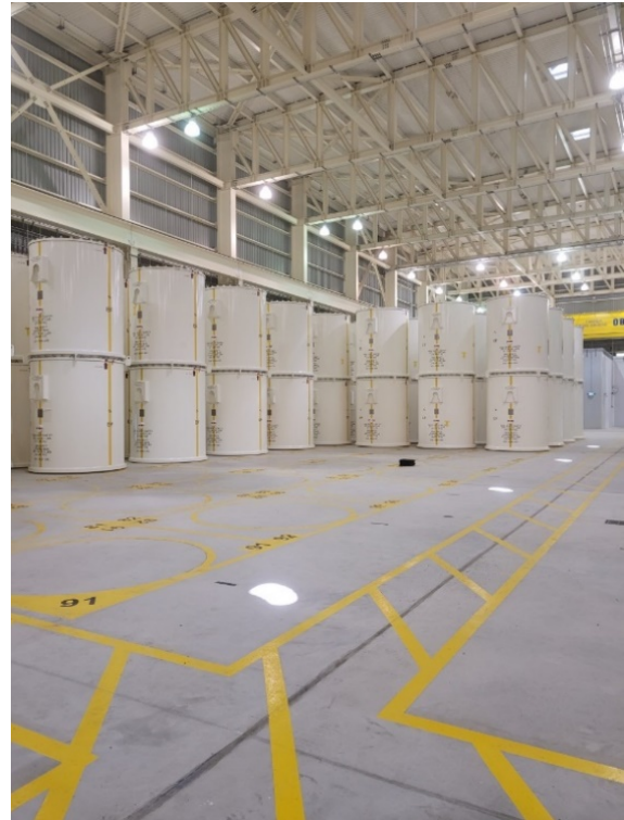
Figure 10: RWC/DSOs in safe storage
