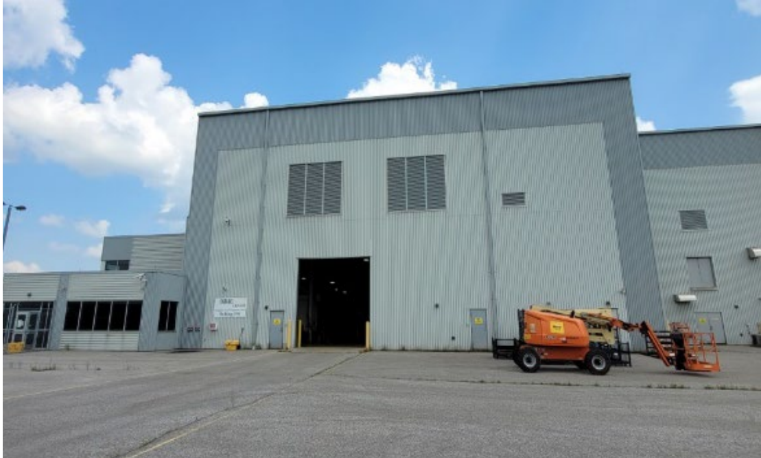
DSC Processing Building
